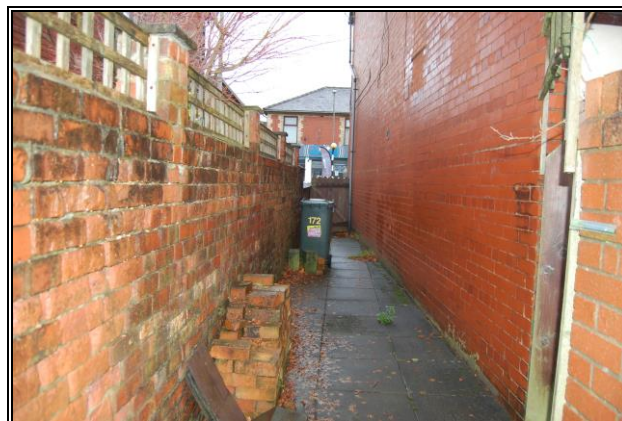
Side Shared Passageway
